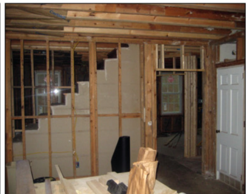
Building under renovation.
