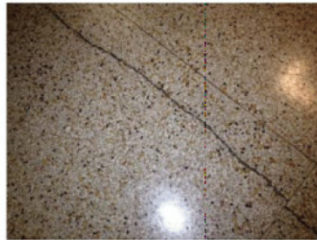
Major floor crack which runs perpendicular to the support wall of the Bell Tower. The Bell Tower also has cracks.
