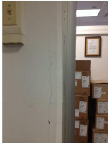
Fourth floor in Computer Department. Photo shows stress crack in plaster around door frame.
