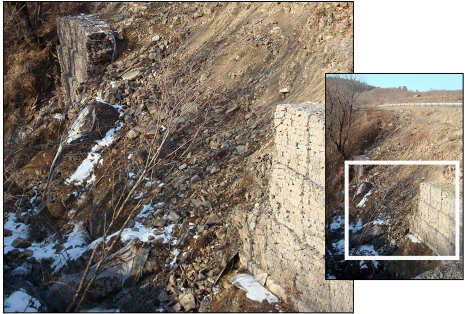
Figure 15: Failed Retaining Wall in Lot 2
