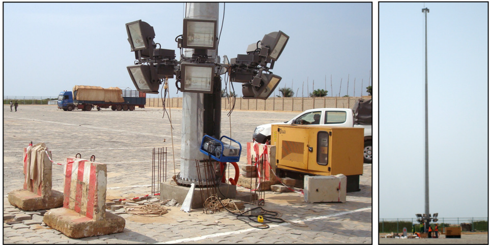
Figure 23: Lighting Pole under Construction
