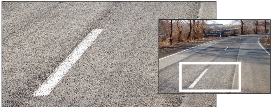
Figure 8: Seal Coat Repair on Center of Road in Lot 4
