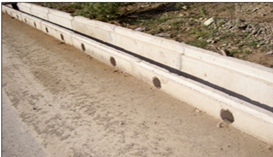
Figure 14: Drainage System Drain Holes Too High to Allow Water to Drain in Lot 3
