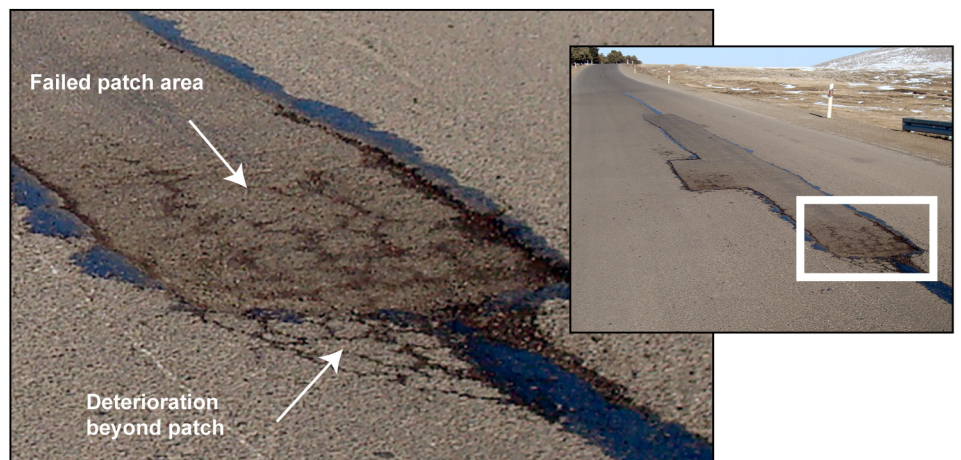
Figure 9: Failed Patch and Continued Deterioration in Lot 3
