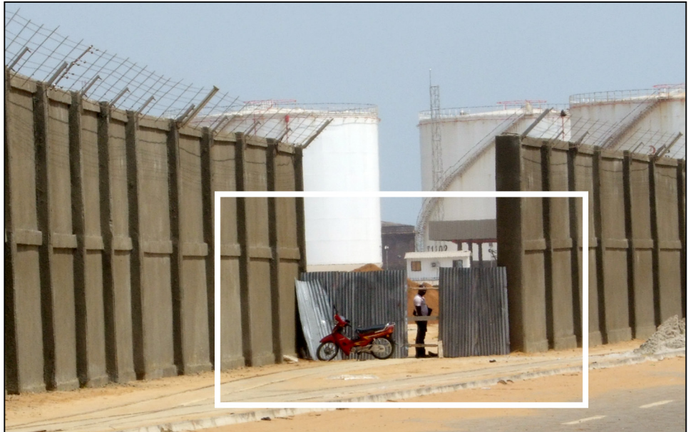
Figure 25: Breach in Boundary Wall
