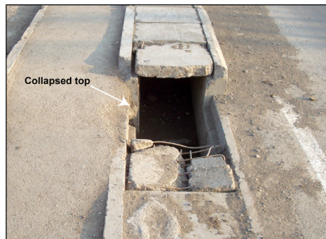
Figure 12: Defective Drain Tops
