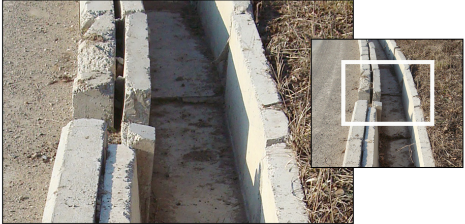
Figure 13: Drainage Channel Construction Defects in Lots 2 and 6i
