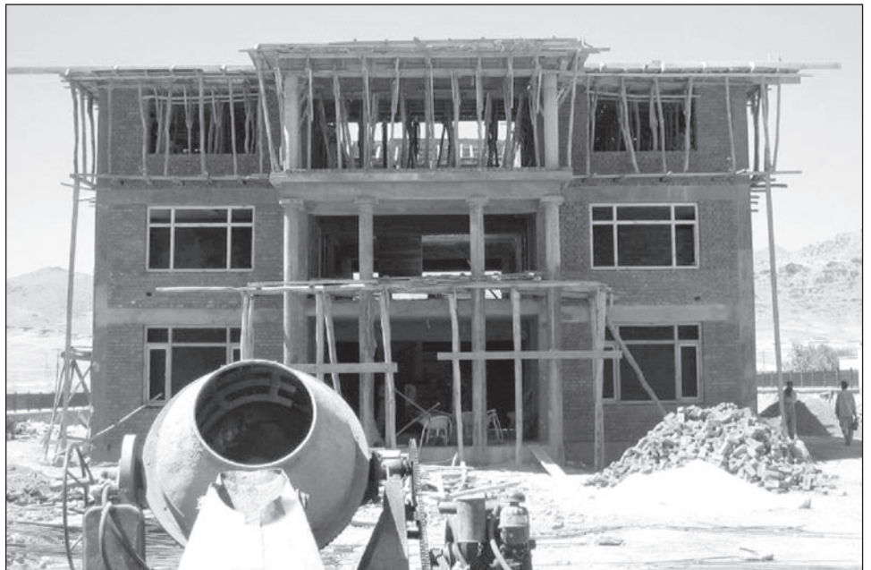
Figure 9: Ministry of Justice Building under Construction in Wardak Province
