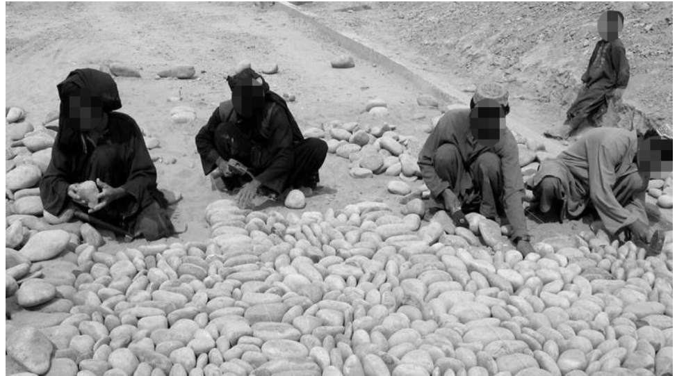
Figure 4: Cash-for-Work Road-Construction Project
