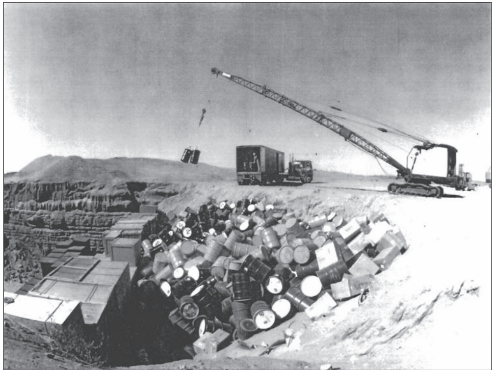
Figure 1: Typical Disposal of Transuranic and Other Wastes in Unlined Trench at the Hanford Site Prior to 1970
