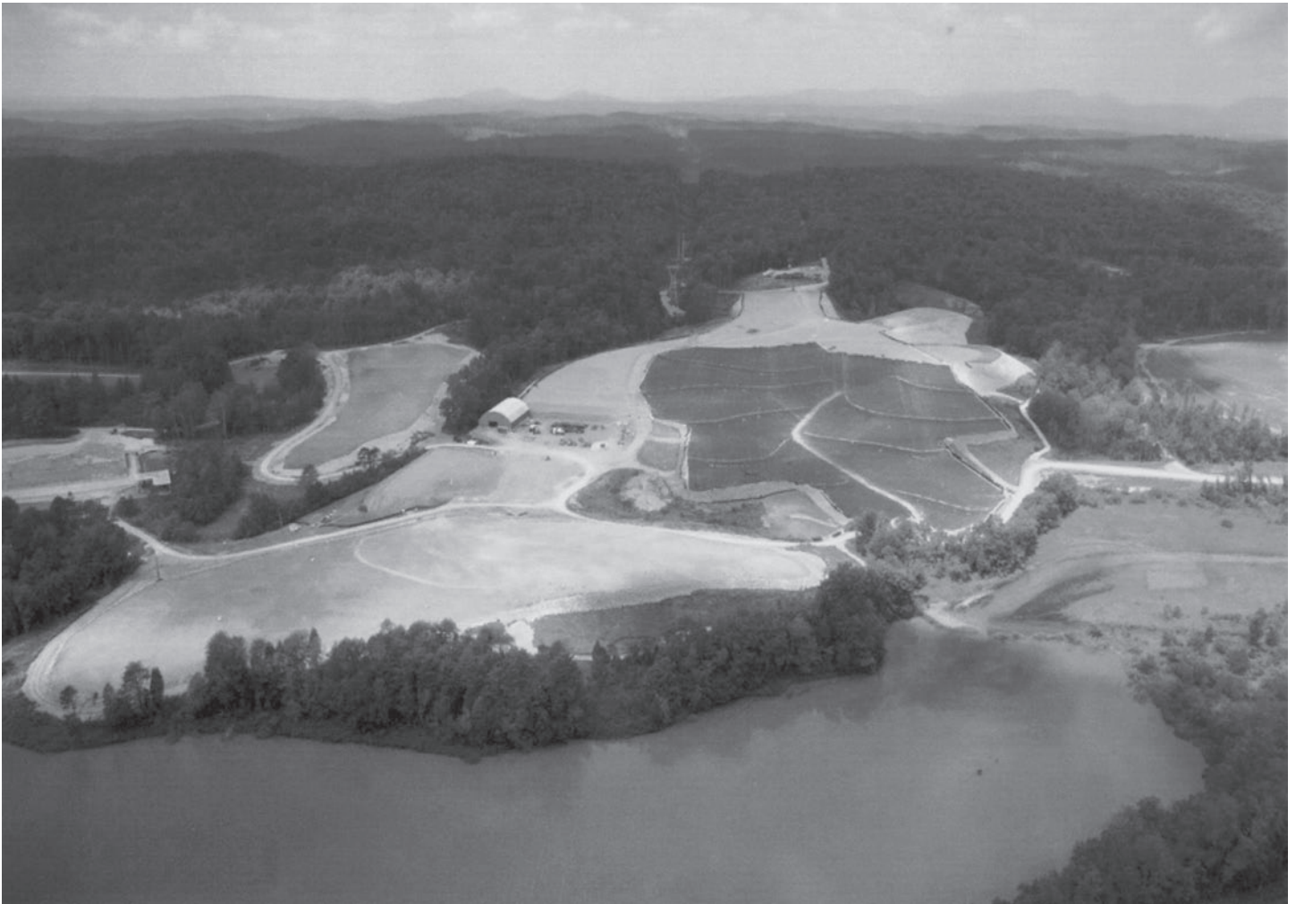
Figure 3: Aerial View of an Engineered Barrier under Construction at Oak Ridge
