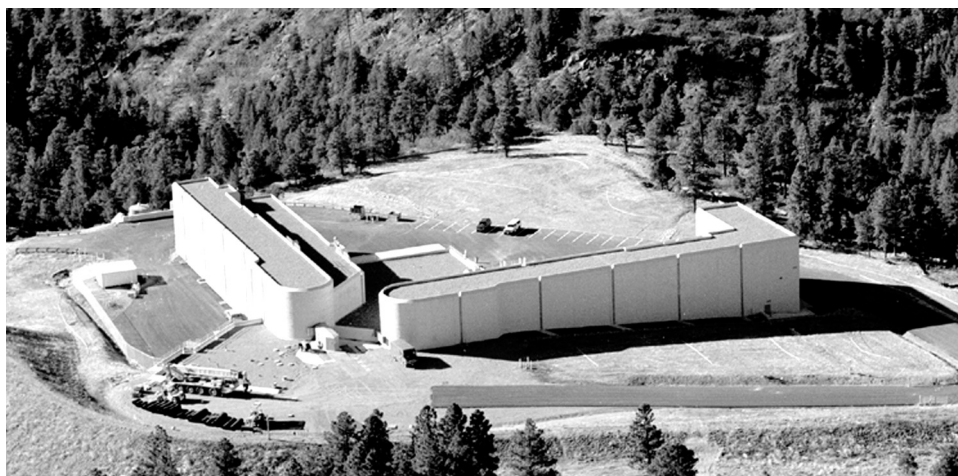
Figure 2: The DARHT Facility at LANL
