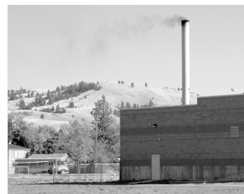
Wood-fired heating facility at rural school.
