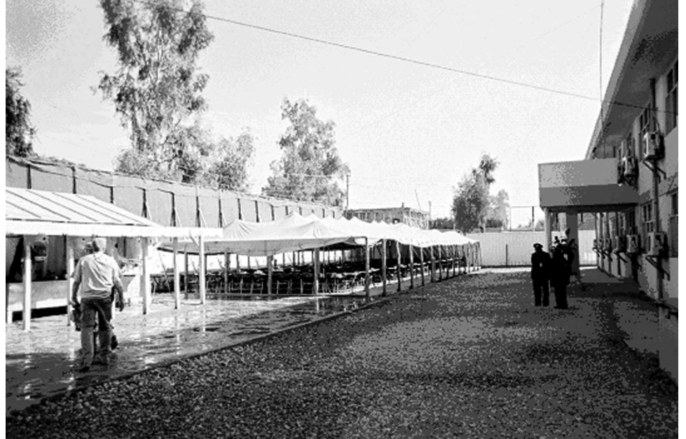
Figure 5: Police Regional Training Center in Jalalabad—Dining Facility and Classroom Building
