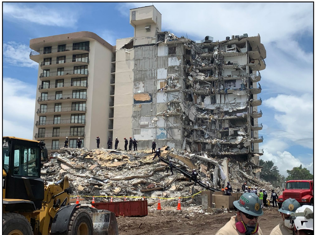
Figure 1: Site of the 2021 Champlain Towers South Collapse in Surfside, Florida
