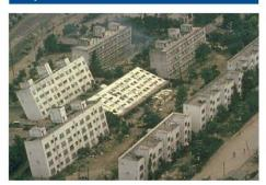
According to USGS, loosely packed, water-logged sediments at or near the ground surface lose their strength in response to strong ground shaking. Liquefaction occurring beneath buildings and other structures can cause major damage during earthquakes because the soil cannot support buildings or other structures. For example, the 1964 Niigata earthquake caused widespread liquefaction in Niigata, Japan which destroyed many buildings.
