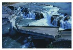
Surface rupture is an offset of the ground surface when a fault ruptures to the Earth's surface. Any structure built across the fault is at risk of being torn apart as the two sides of the fault slip past each other. For example, the 1999 Chi Chi, Taiwan earthquake raised the upper stream 15 to 20 feet creating a new waterfall.
