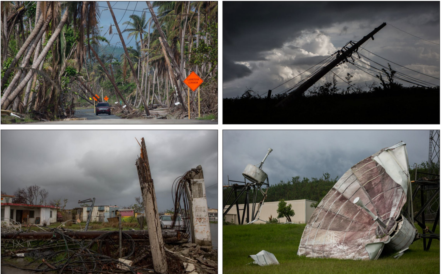
Figure 3: Damaged Power Lines and Satellite Dish in Puerto Rico After Hurricane Maria in November 2017
