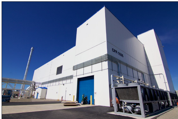
Figure 2: Exterior of the Department of Energy’s (DOE) Integrated Waste Treatment Unit at Idaho National Laboratory
