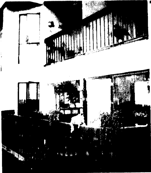
BALCONY/PATIO, WITH IRON ROD RAILING
