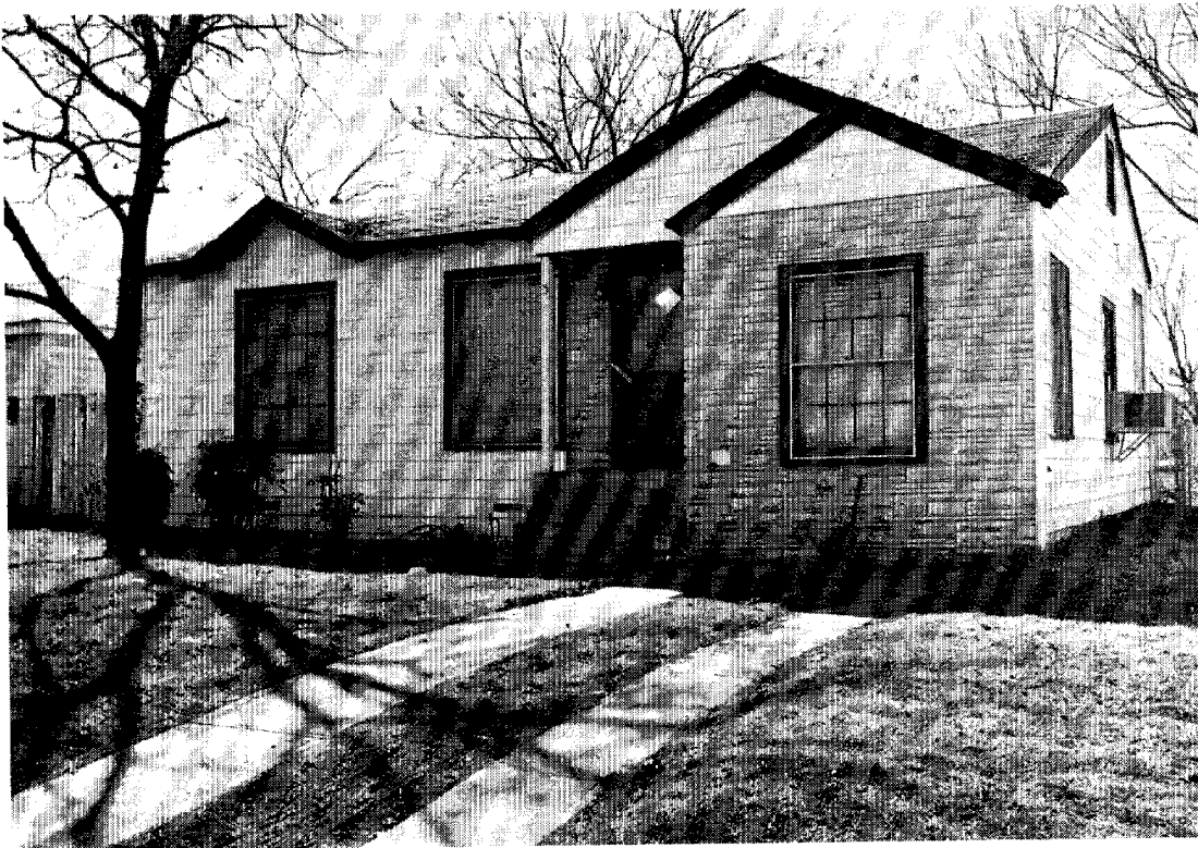
SAME HOUSE AFTER REHABILITATION.
