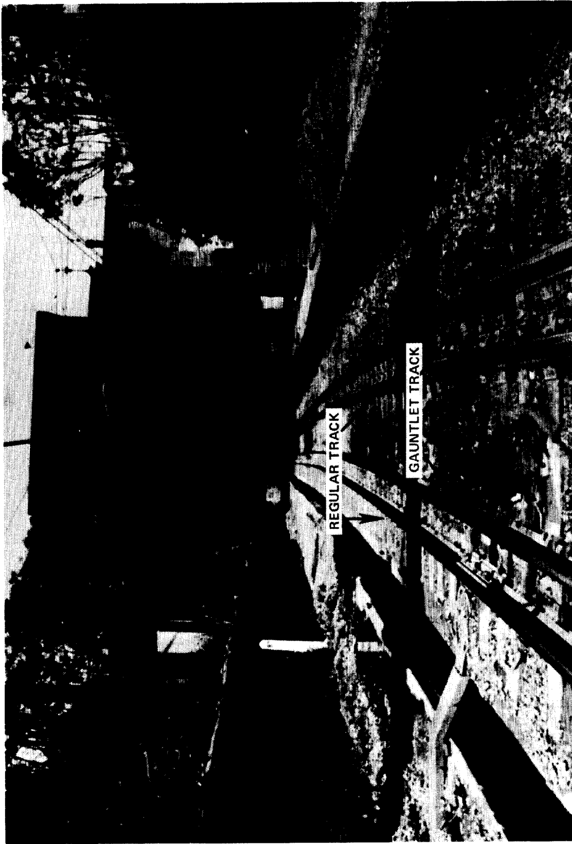
VIEW OF THE B&P TUNNEL IN BALTIMORE SHOWING THE GAUNTLET TRACK
