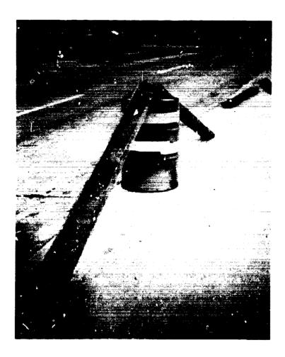
Heavy steel forms were used extensively at one project to anchor metal drums in the manner shown above.
