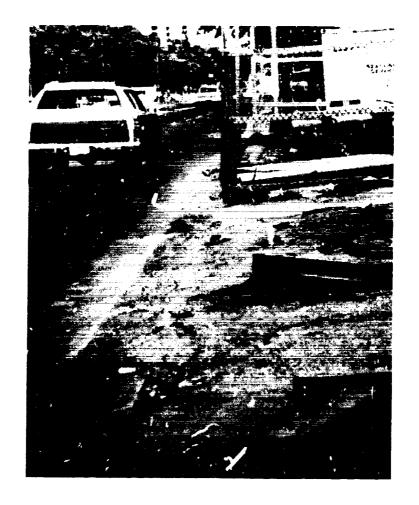
The fenced-in area contained various sizes of water and sewage pipes and was flush with the edge of the traffic lane. Lack of reflective markings on the fence caused a hazardous condition at night.
