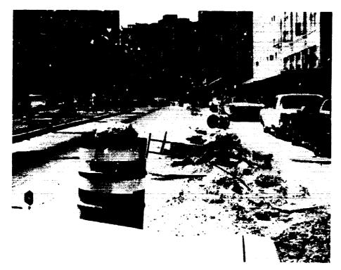
A piece of concrete was used to stablize this drum.
