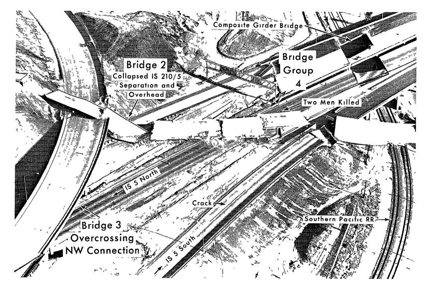
Freeway damage caused by the San Fernando, California, earthquake of February 9, 1971 Two men in a truck lost their lives as a result of the collapse of the freeway separation and overhead (Los Angeles Times Photo)
