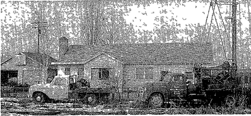
Well Rig on Location
