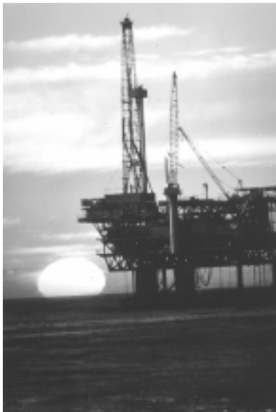
Offshore Oil Platform
