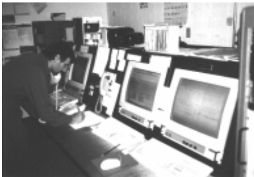
Control Center for Offshore Oil Platform Monitoring and Control
