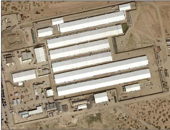
Aerial photo of Camp East Montana
