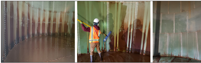
Before water storage tank cleaning
