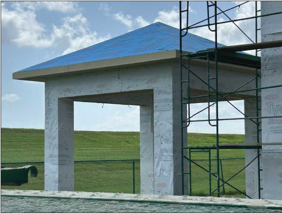
Figure 14: A Home in Louisiana with a Sealed Roof Deck—A Required Feature for Roofs Built to the FORTIFIED Construction Standard
