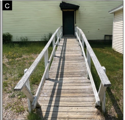
Image C: The only wheelchair accessible entrance into the school.
