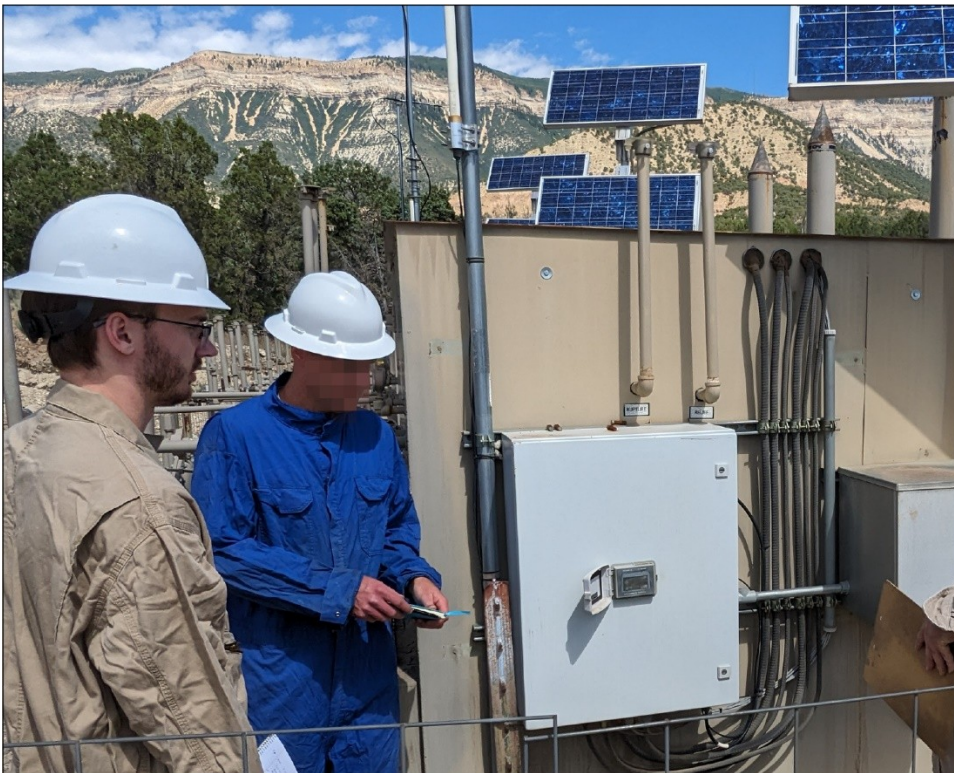
Figure 2: Flow Computer Capturing Data About Natural Gas Production at an Oil and Gas Well on Federal Land
