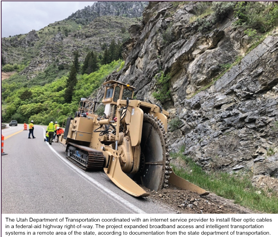
Figure 1: Example of Excavation to Install Fiber Optic Cables in a Federal-Aid Highway Right-of-Way
