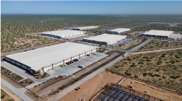
Image showing commercial warehouse space in Santa Teresa, New Mexico.
