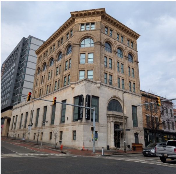
GAO site visit observations in Baltimore, Maryland.
