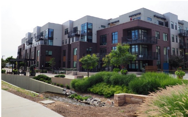
GAO site visit observations in Boulder, Colorado.
