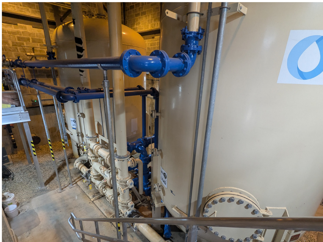
Figure 10: Brookhaven National Laboratory Building Originally Slated for Demolition Was Repurposed to Treat Per- and Polyfluoroalkyl Substances in Groundwater with Granular Activated Carbon Filters
