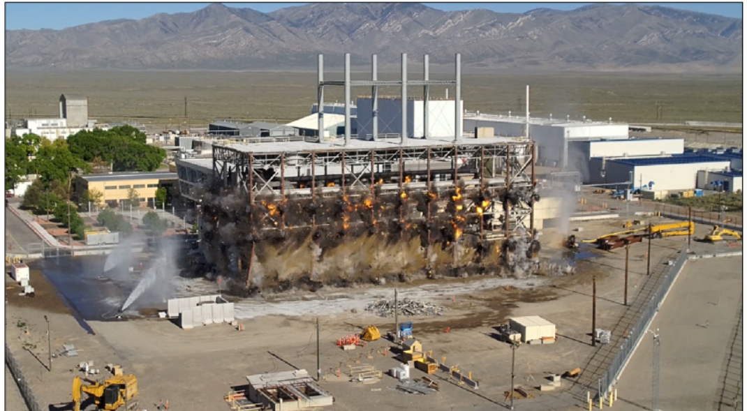
Figure 1: Demolition of the Submarine First Generation Westinghouse (S1W) Nuclear Propulsion Prototype Facility at a DOE Office of Naval Reactors Site in Idaho
