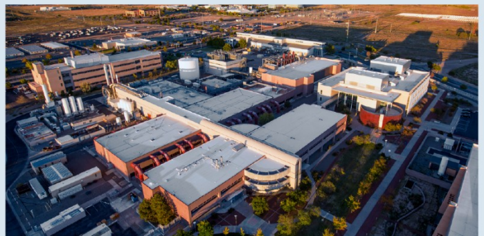
Current MESA facility complex.
