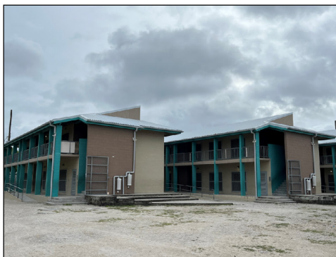
Completed school buildings.
