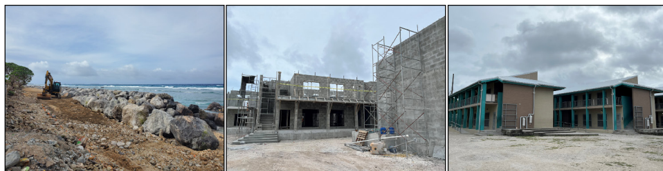
Construction of sea wall.
