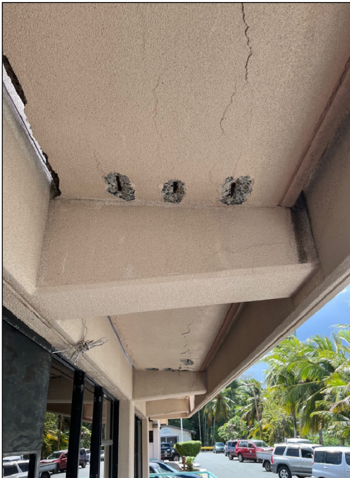
Visible water damage, exposed and rusted rebar, and cracks at Palau hospital.
