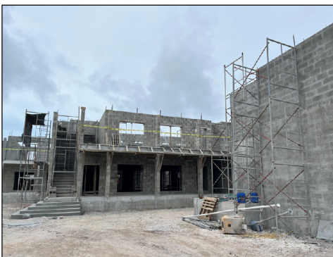
Construction of new classrooms.
