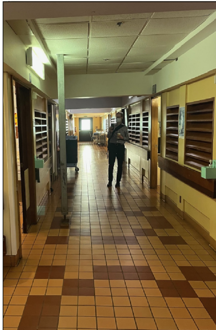
Ceiling supported by pole in hospital corridor.
