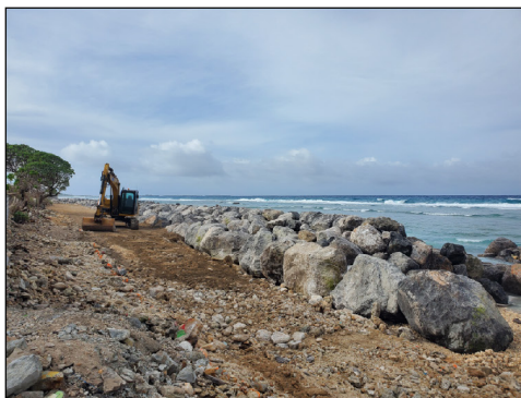
Construction of sea wall.
