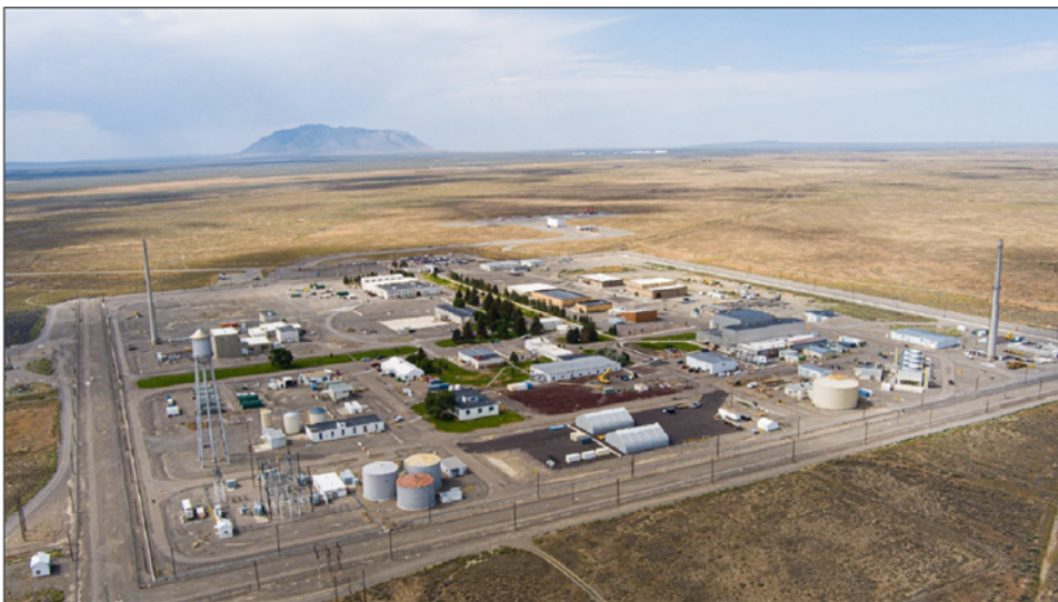
Figure 1: Advanced Test Reactor Complex, Idaho National Laboratory
