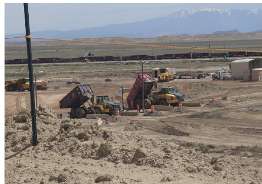
Two trucks unloading containers of tailings at the Crescent Junction Disposal Site.
