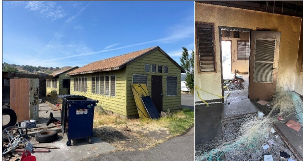
Figure 6: Example of Existing Infrastructure That CRITFC Plans to Improve at the Lone Pine Fishing Access Site on the Columbia River
