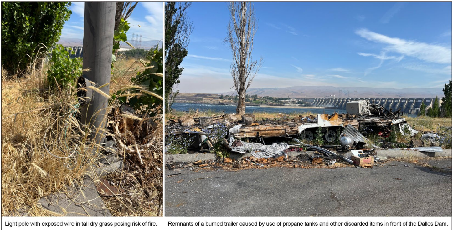
Figure 7: Examples of Fire Safety Hazards at Columbia River Fishing Access Sites
