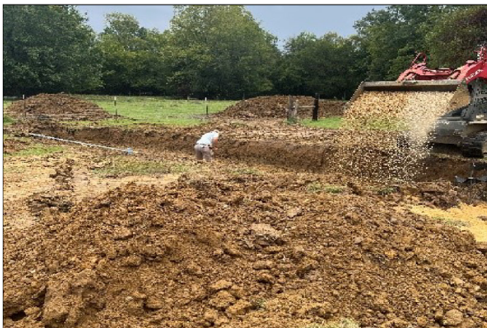
Figure 7: Installation of a Septic System at a Rural Home in Alabama
