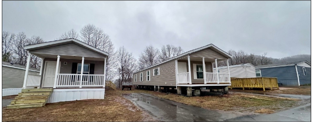
Figure 6: Federal Emergency Management Agency Manufactured Housing Units in North Carolina After Hurricane Helene
