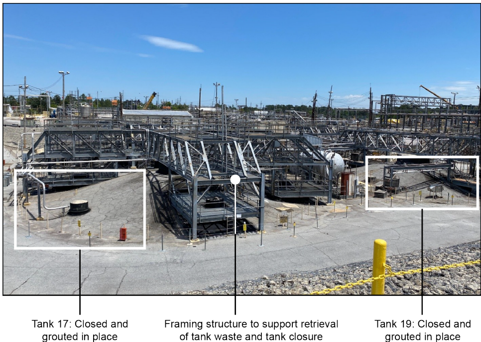
Figure 4: Grouted Waste Tanks and Associated Infrastructure at the Savannah River Site’s F Tank Farm, May 2025
