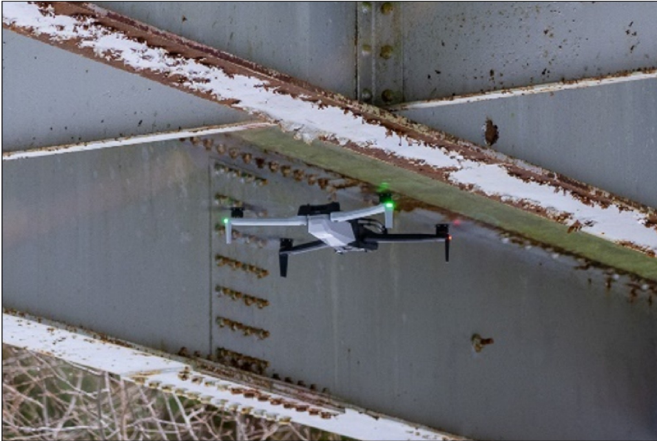
Figure 5: Alaska Drone Inspecting a Bridge for Corrosion
