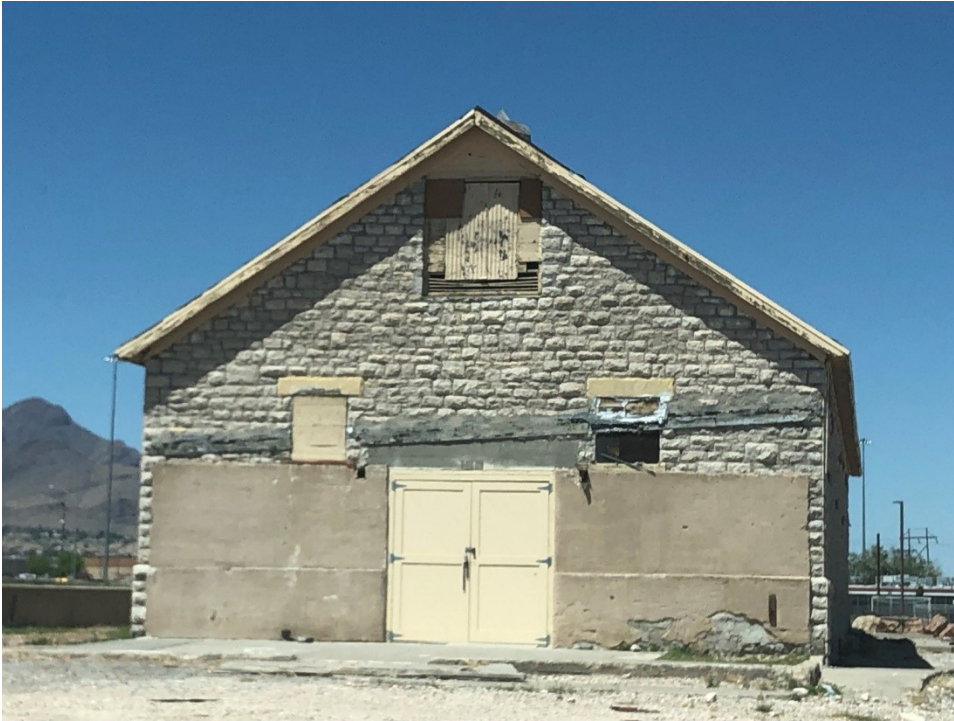
Figure 4: Vacant Historic Building at Fort Bliss, Texas
