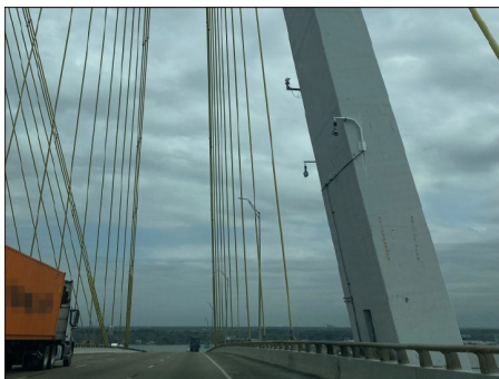
Surveillance cameras on a bridge
