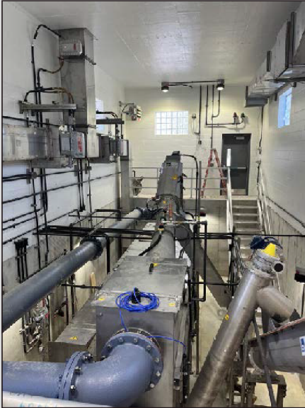
Wastewater Treatment Plant Improvements Partially Funded by USDA Loan
