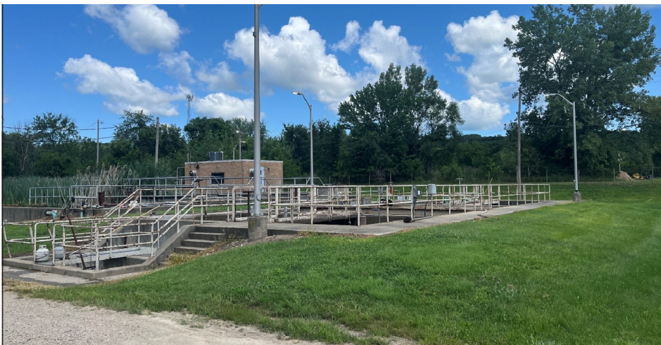
Figure 6: Wastewater Treatment Plant in DePue, IL
