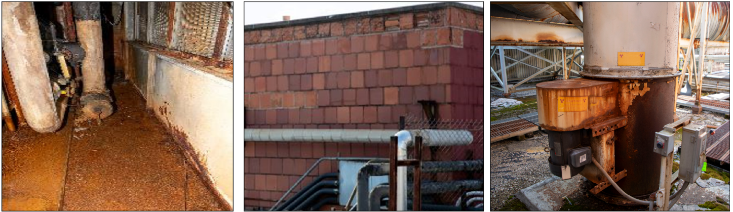
Figure 4: Examples of Structural Degradation of Uranium Processing and Support Buildings
