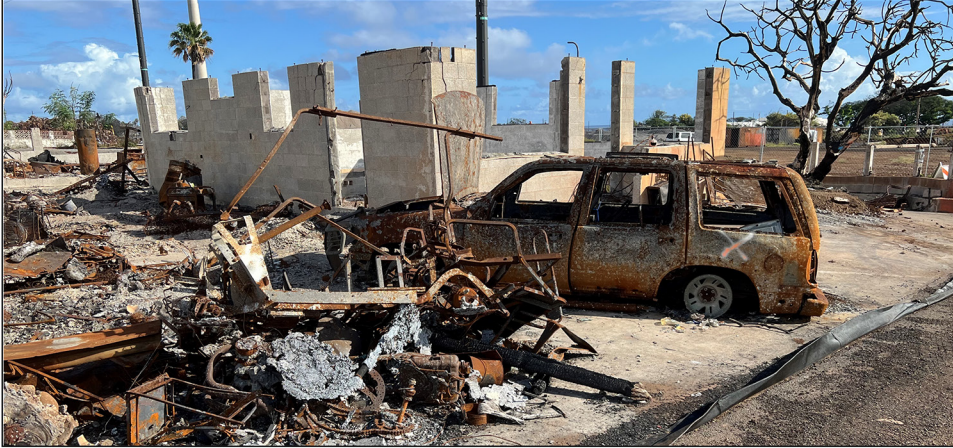
Source: Damage at site of Maui wildfires; GAO (photo). | GAO-25-107136
