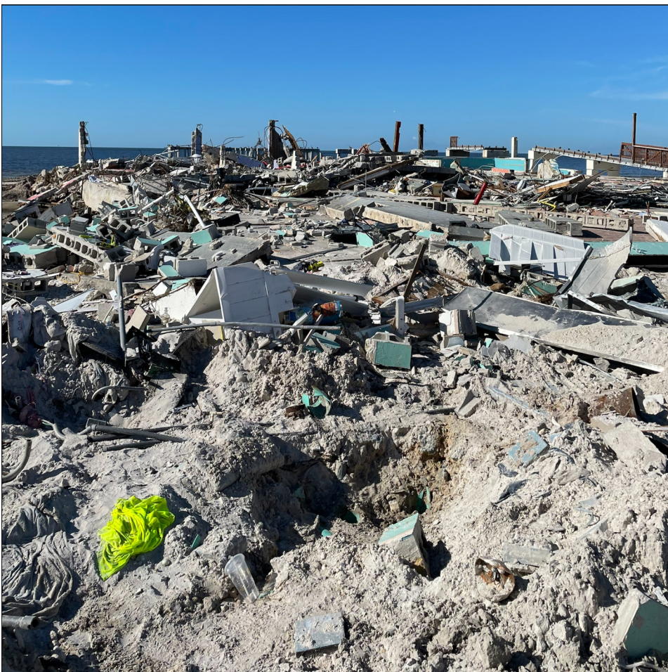
Figure 10: Hurricane Ian Damage
