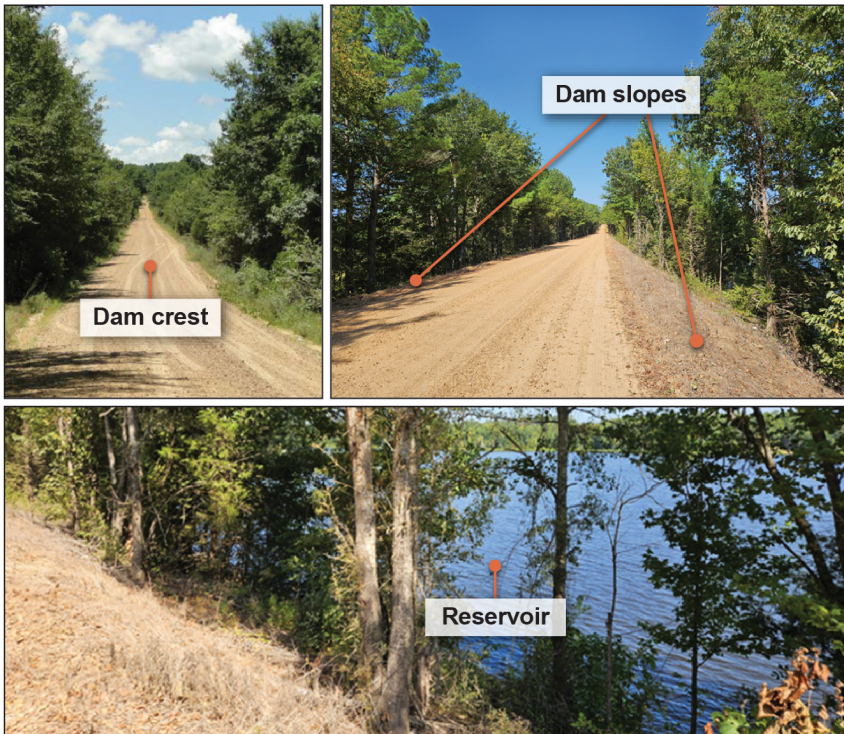
Figure 4: Embankment of Natural Resources Conservation Service Watershed Dam with Heavy Vegetation, Mississippi, 2017 (top left) and 2024 (top right and bottom)
