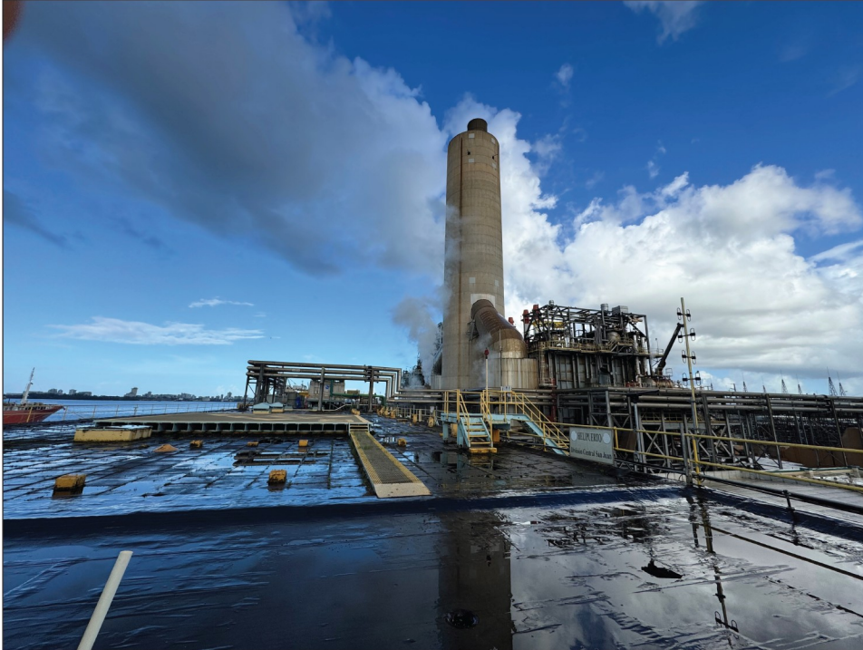
Figure 2: FEMA Public Assistance Project Using CDBG-DR Funds for the Cost-Share Requirement: San Juan Central Generation Station
