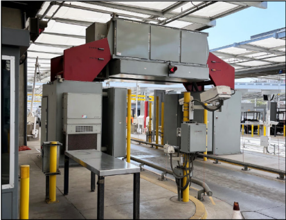
Z-portals scan passenger vehicles and buses.
