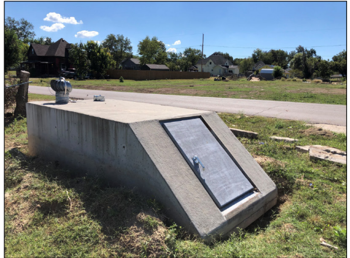
Residential safe room in Sulphur, Oklahoma
