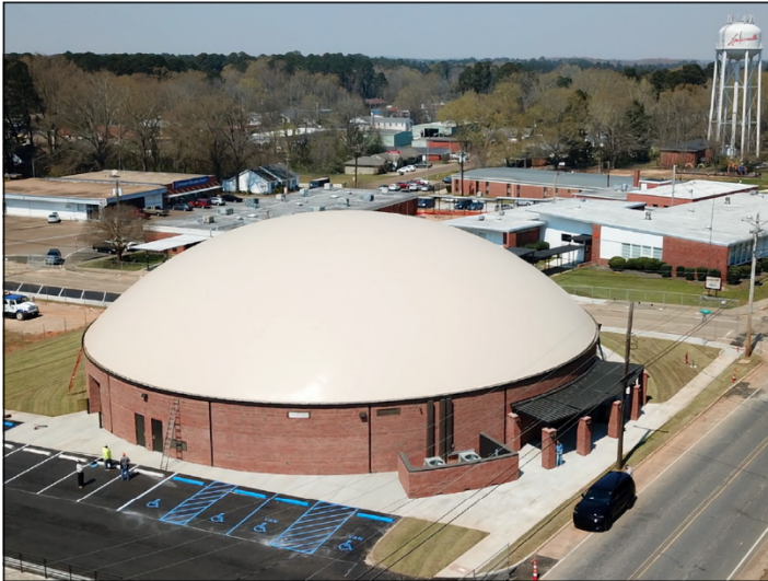
Community safe room in Louisville, Mississippi
