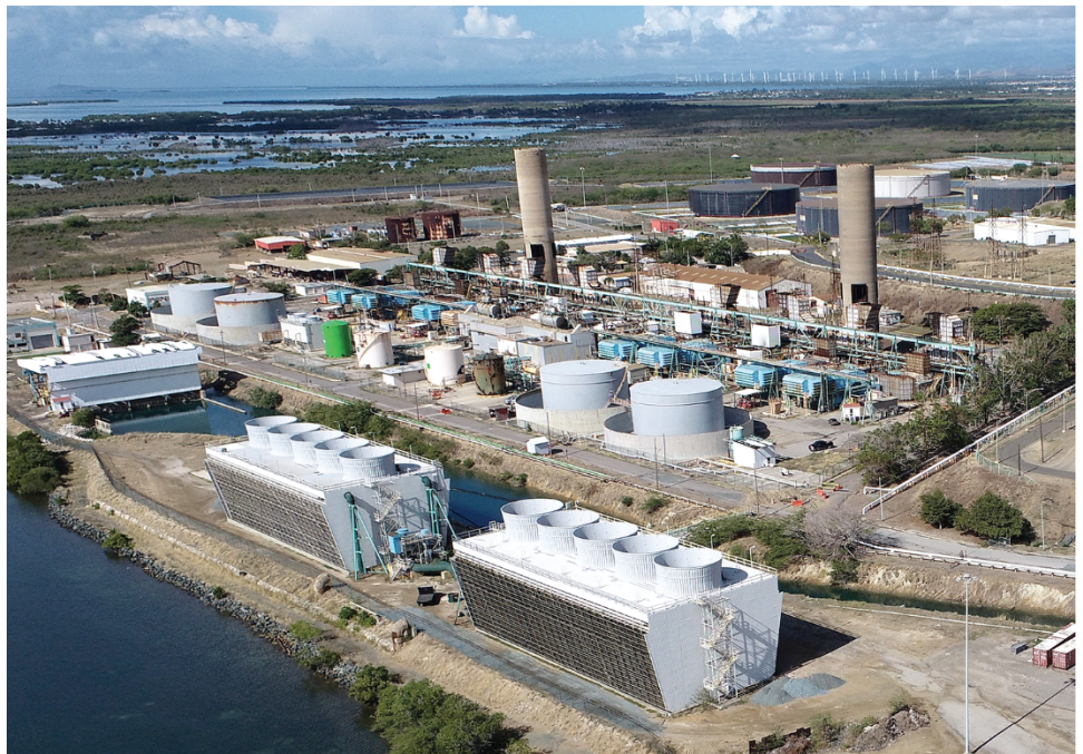
Figure 4: Aguirre Power Generating Plant in Salinas, Puerto Rico
