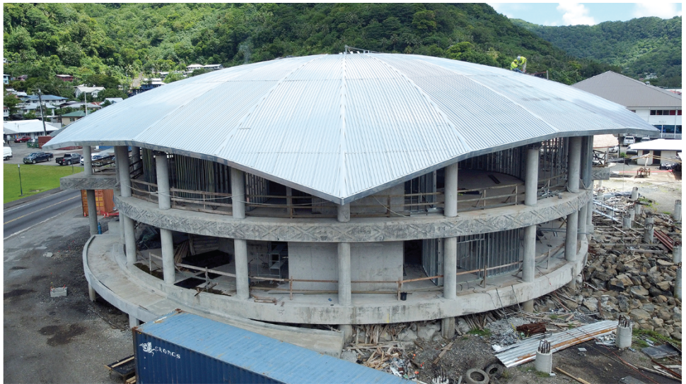
Figure 18: American Samoa Fono Legislature Building, Under Construction
