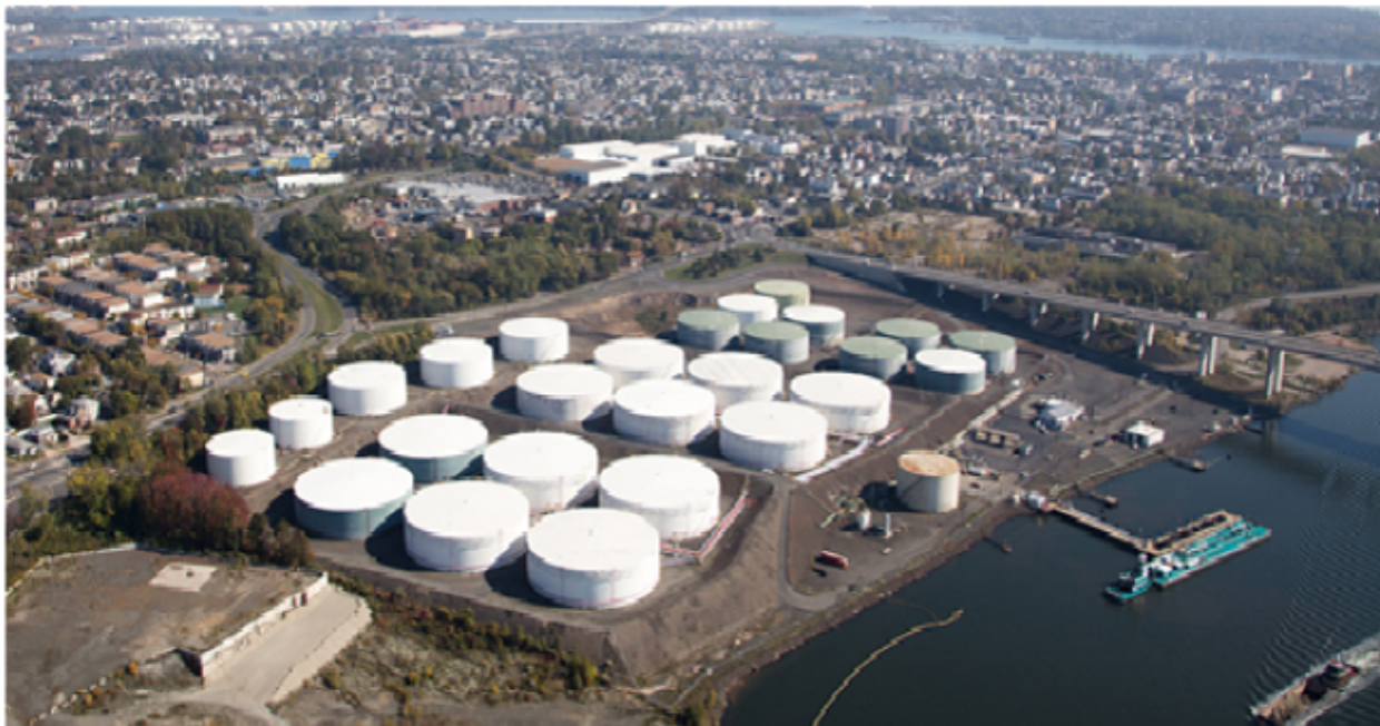
Figure 2: Storage Tanks Holding Northeast Gasoline Supply Reserve and Commercial Supplies at Raritan Bay Facility in New Jersey
