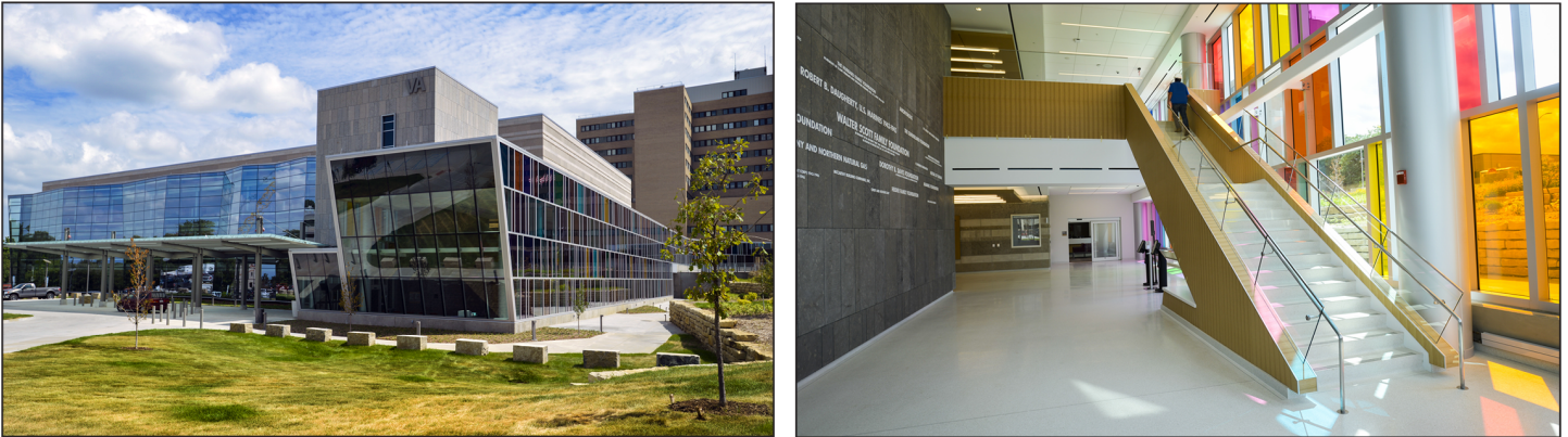
Figure 1: Department of Veterans Affairs' (VA) Ambulatory Care Center in Omaha, NE—Exterior and Interior Views
