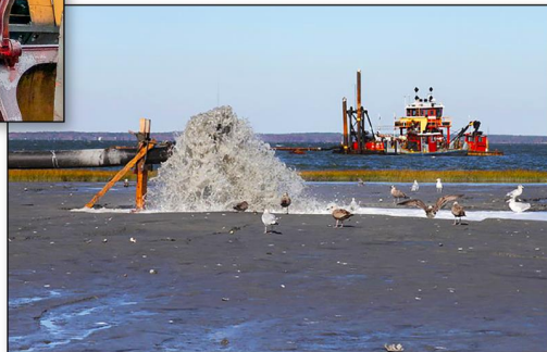
Step 2: Sand is pumped onto shore through a pipe.
