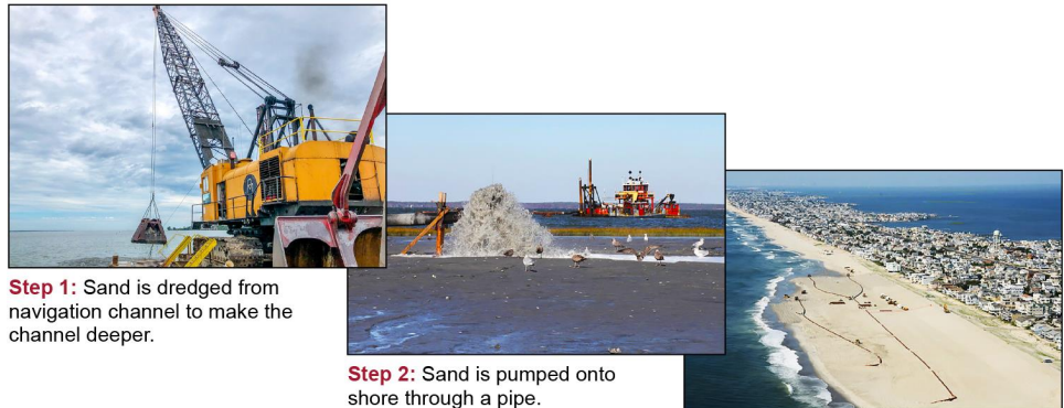
Step 3: Sand is deposited on the shore to replace sand that has been eroded or to build dunes on the beaches.
